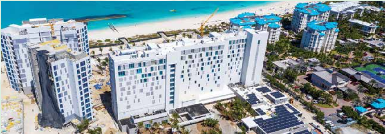
The Ritz-Carlton Turks and Caicos is FortisTCI's 10th Utility Owned Renewable Energy (UORE) partner. A 210.6kW solar PV system has been installed on the roof of the resort's casino and restaurant, and commissioned into service.
