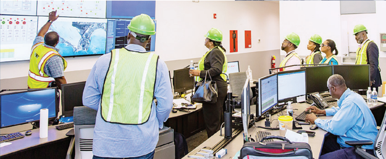
Members of the TCl Immigration Board get a close up view of FortisTCl's state-of-the-art operators room, with Alvejes Desir (left).
